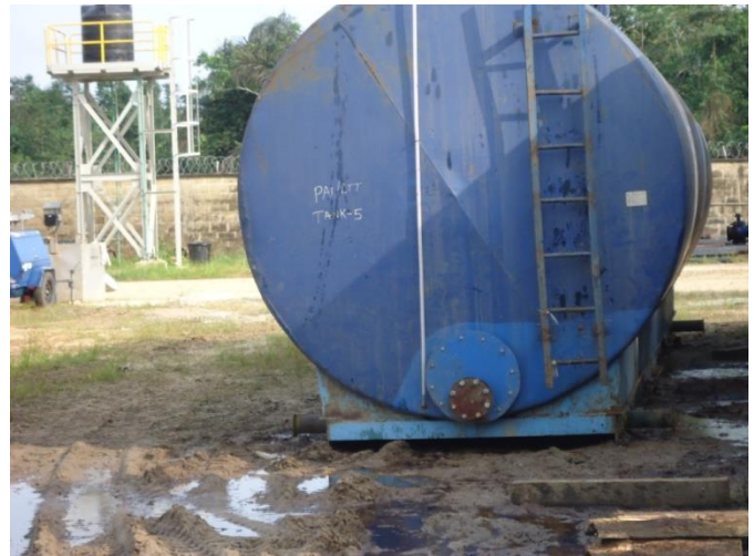
6-7: This empty space (Pic6) shows that Tank 5 that had a ruptured flange which caused spill has been isolated (Pic7)
