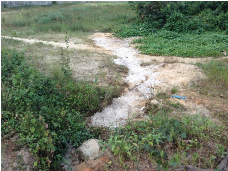
12-13: Spill covered with Sand to contain the Spill sighted (Pic12 and 13)
